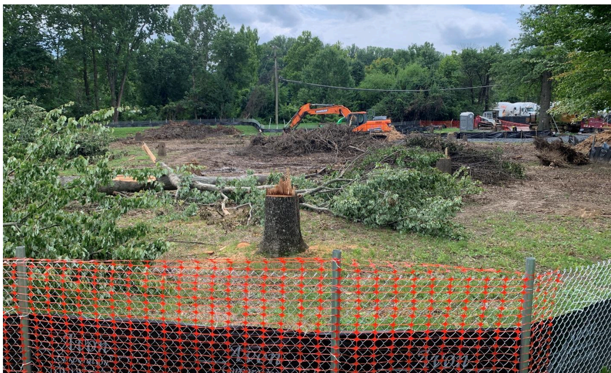
Daunting view of the first stage of Gateway Park project
